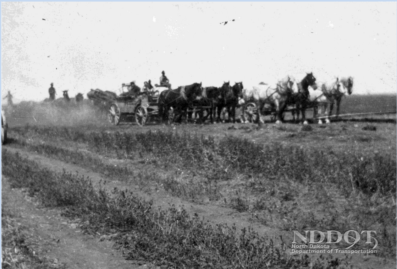
This 1920s photograph shows earth moving and hauling for a roadbed.
